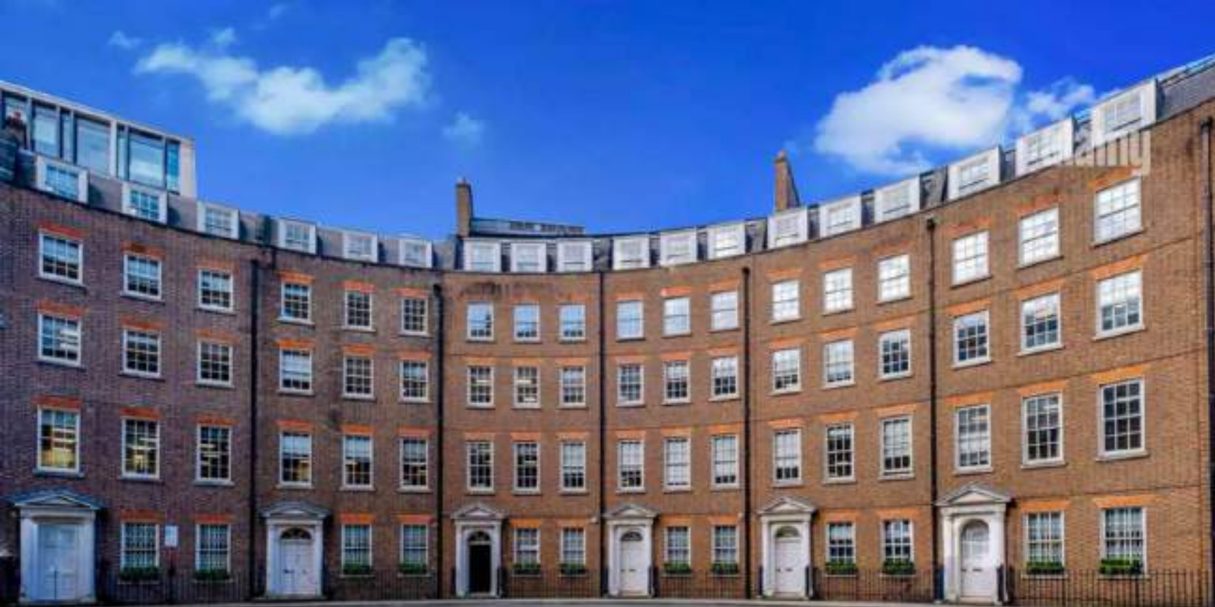
Tower Apartments in the Crescent
